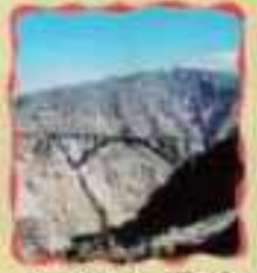
Chamb Bridge—World's Highest Railway Bridge - p. 77
